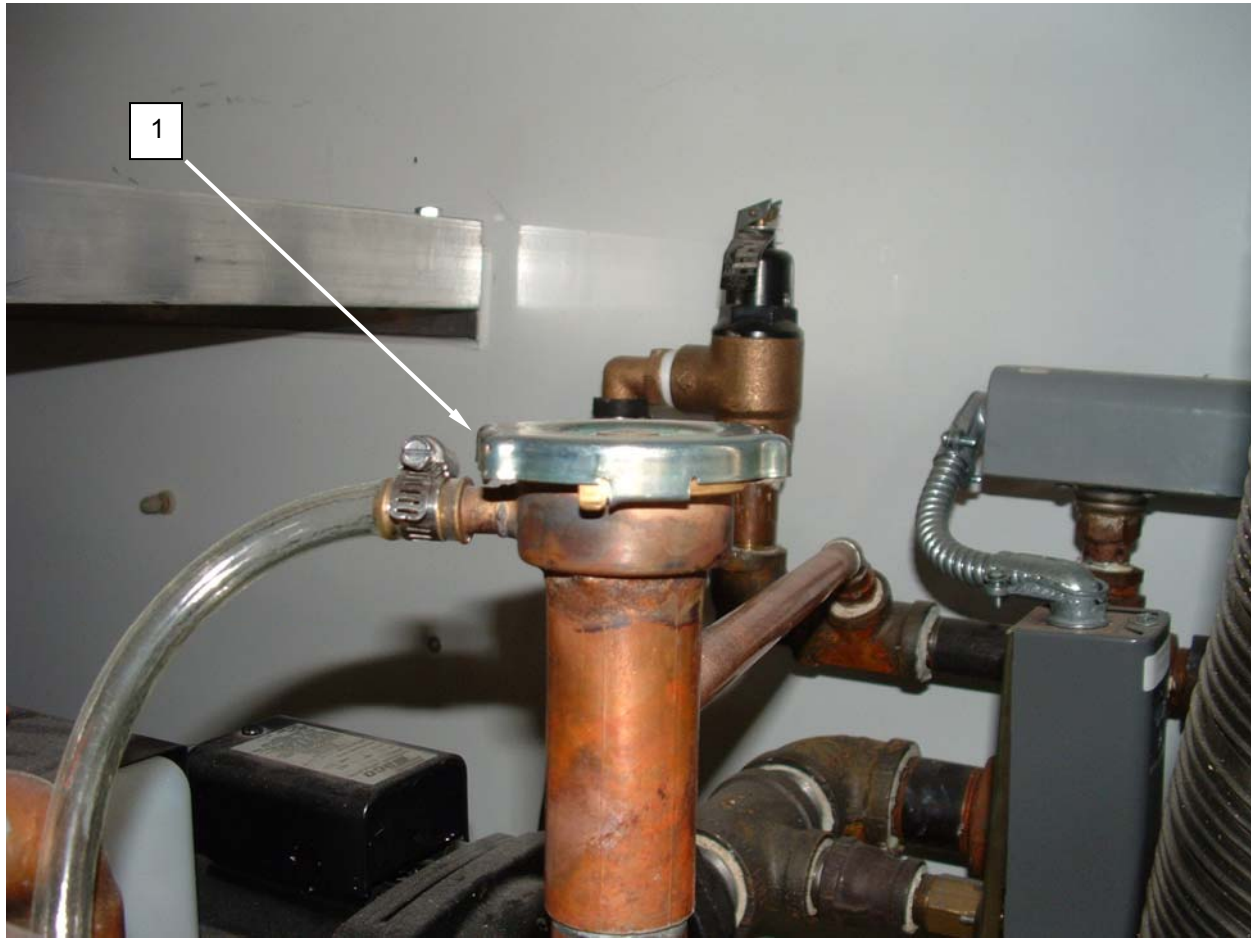
Figure 1. Replace the Pressure Regulating Cap.
