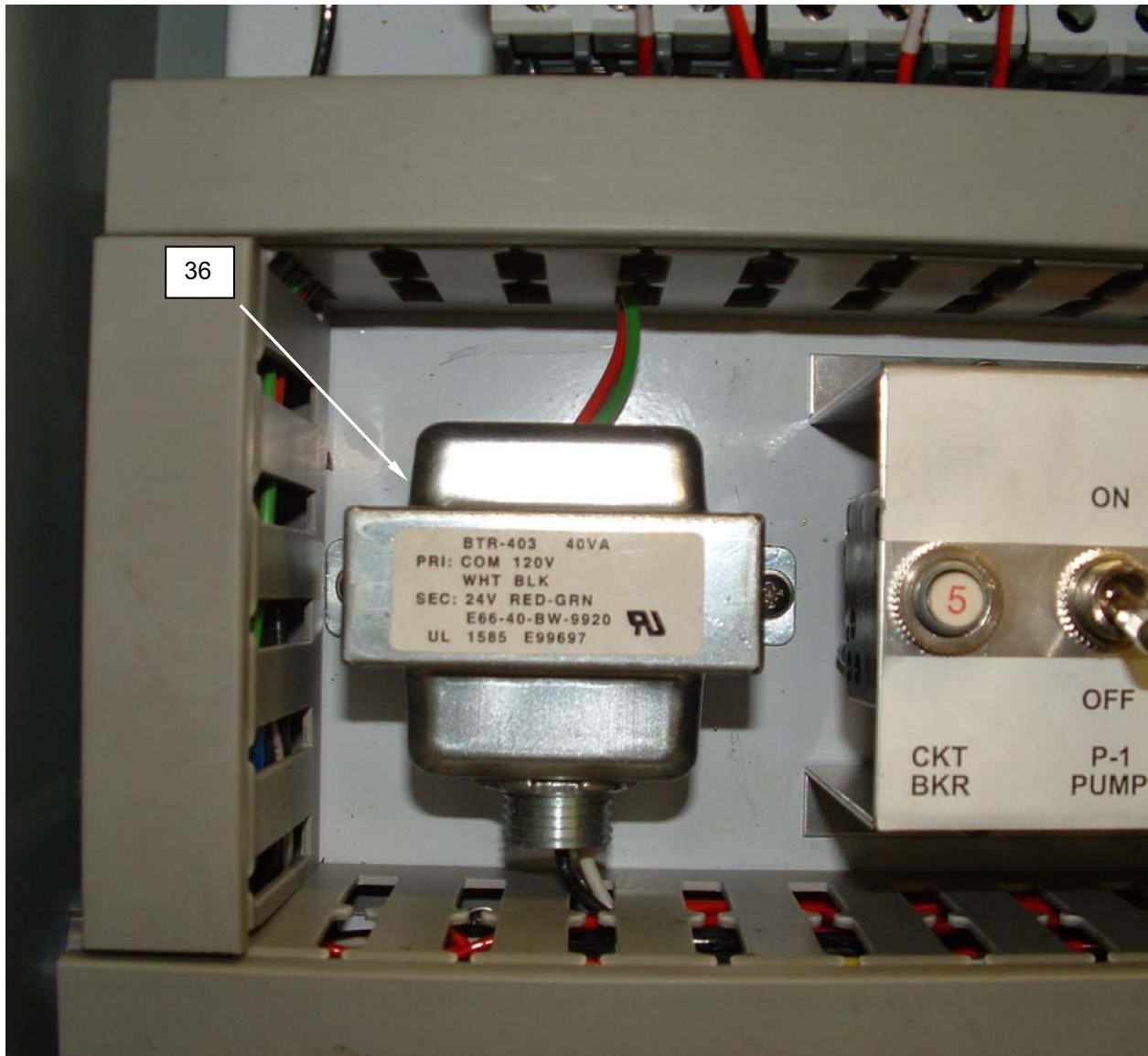
Figure 19. Test the Control Transformer.
