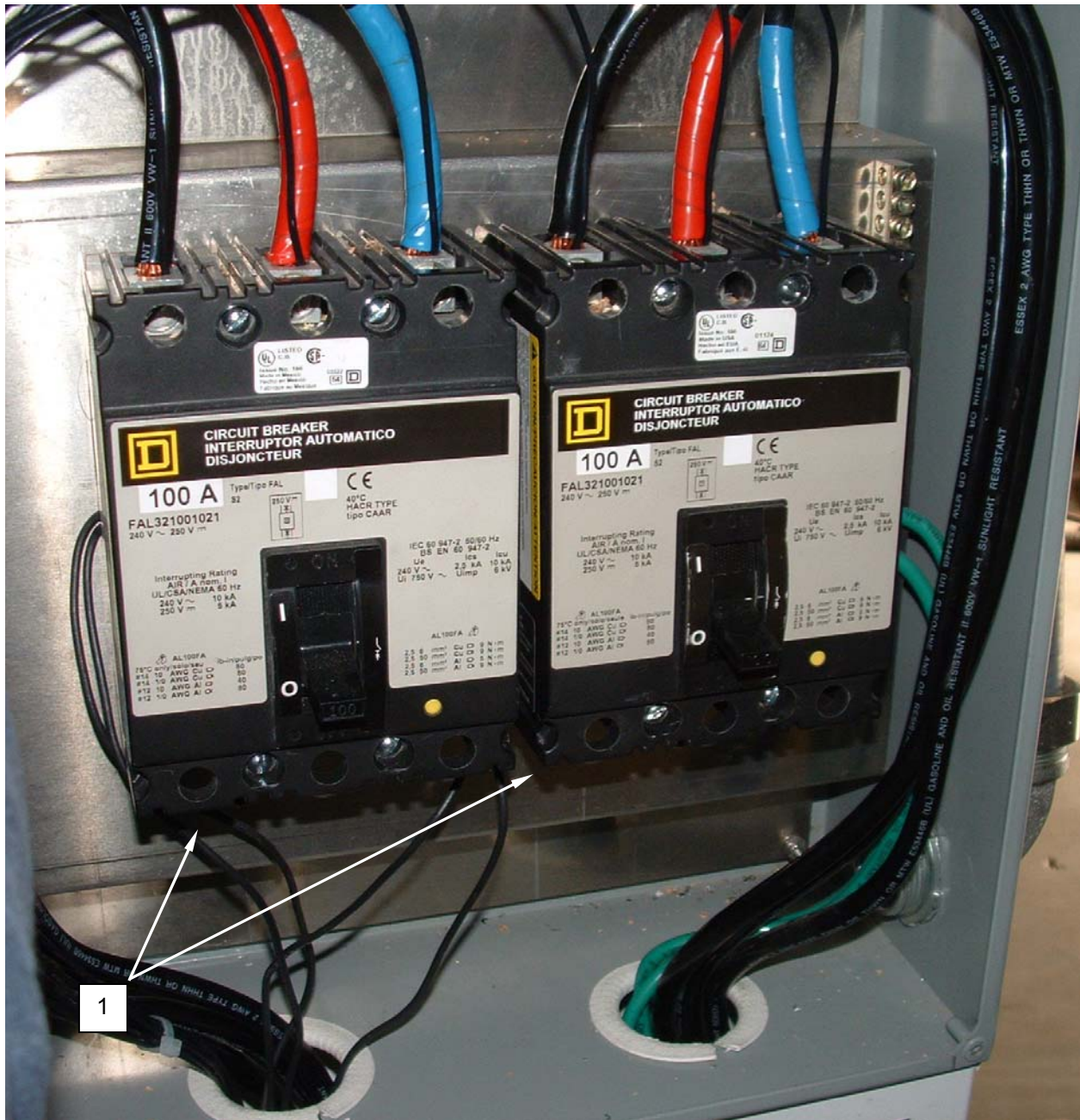
Figure 8. Replace Circuit Breakers – Dryer Panel.
