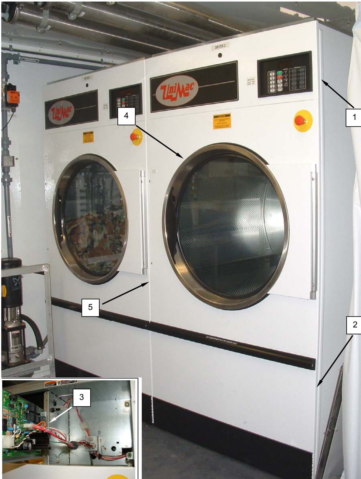
Figure 3. Replace the Dryer Emergency Stop Switch.
