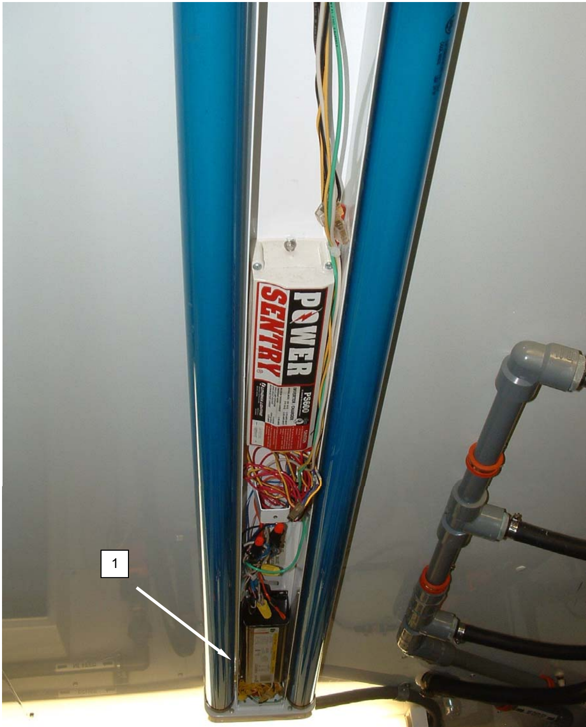
Figure 1. Replace the Ballast.
