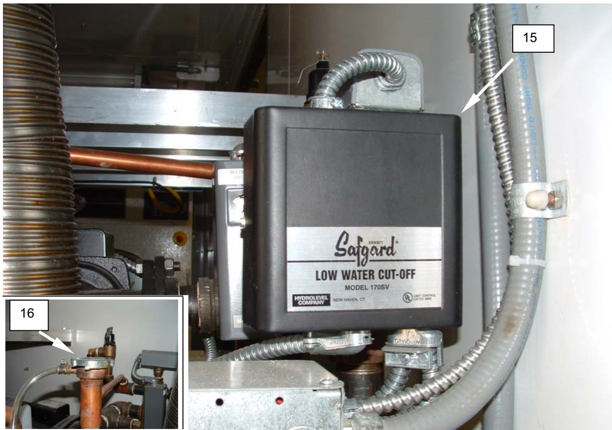
Figure 5. Test the Low Water Cutoff.
