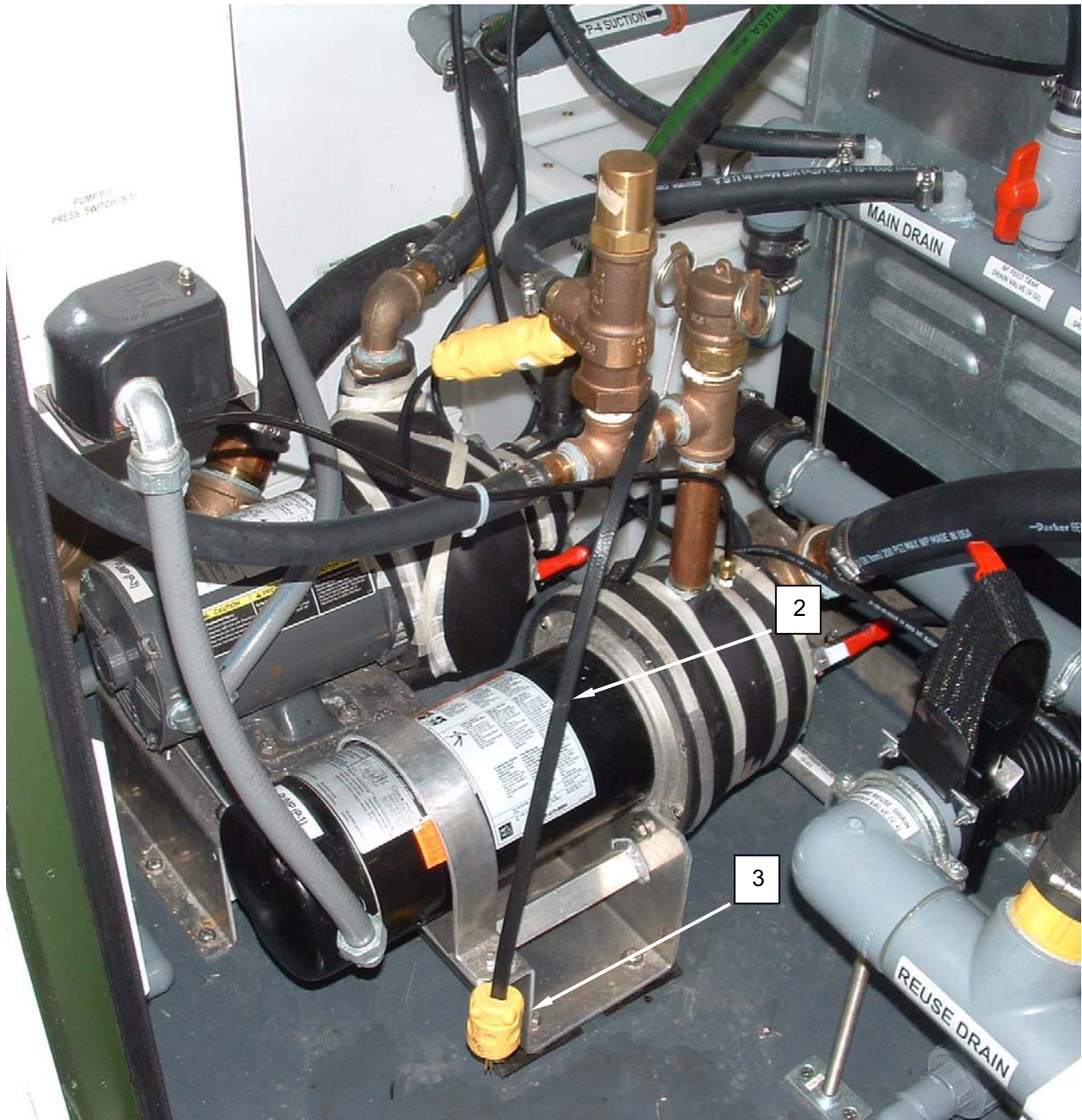
Figure 2. Test the Heat Tapes.
