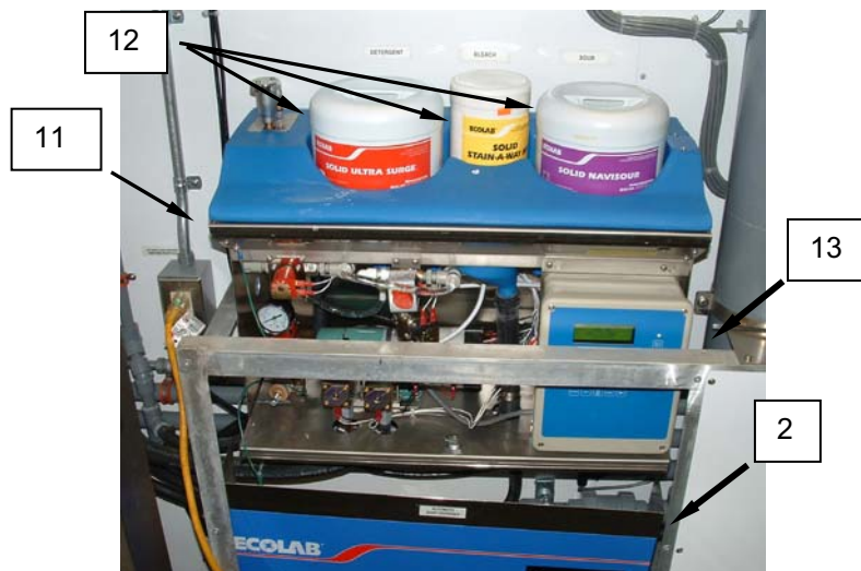
Figure 8. Replace the Automatic Soap Dispenser.
