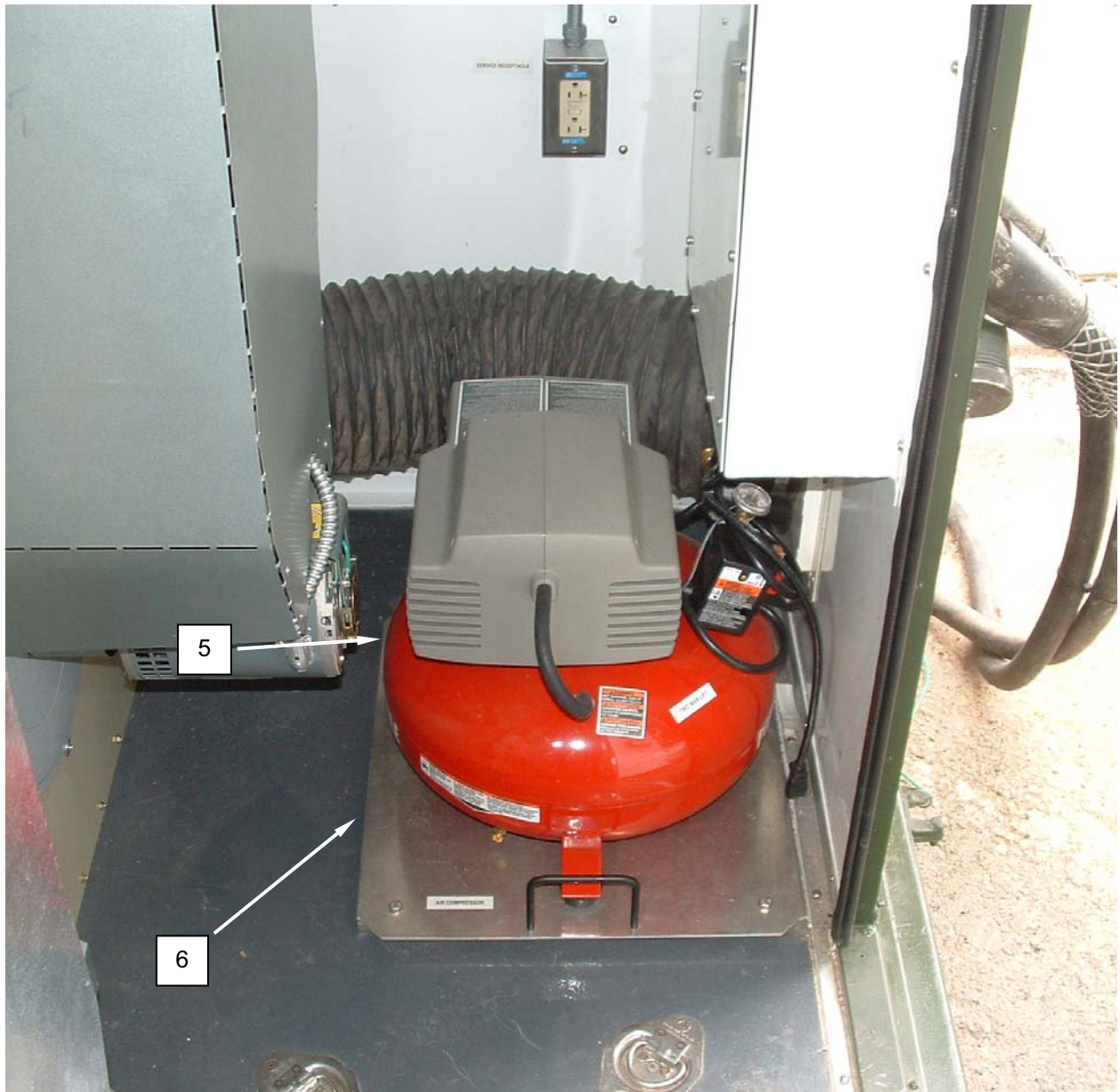
Figure 4. Replace the Air Compressor.
