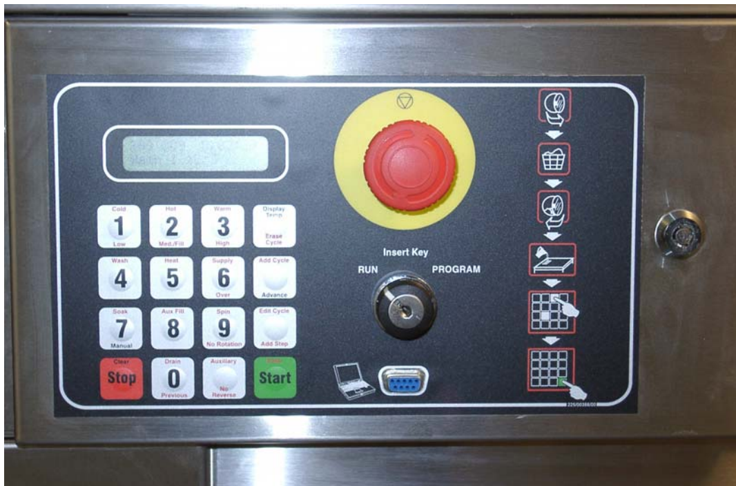
Figure 1. Test the Variable Frequency Drive.
