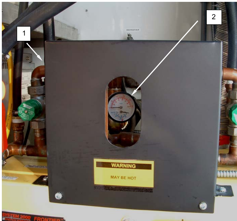
Figure 1. Replace the Pressure-Temperature Gauge.
