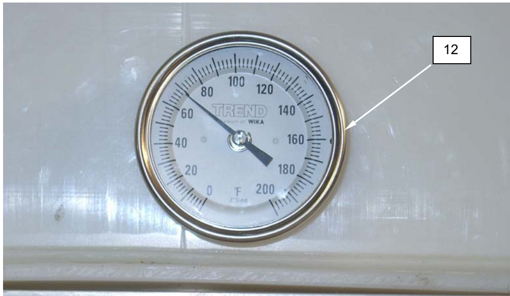
Figure 4. Replace the Reuse Water Temperature Gauge.
