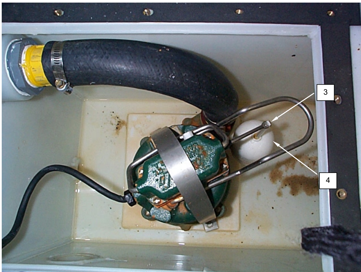
Figure 3. Replace the Drainage Tank Pump Float.
