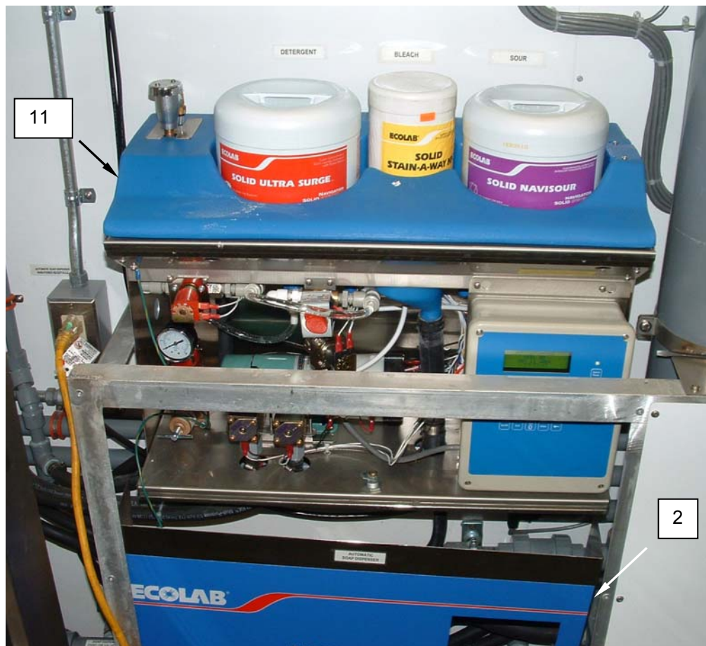
Figure 11. Replace the Automatic Soap Dispenser.
