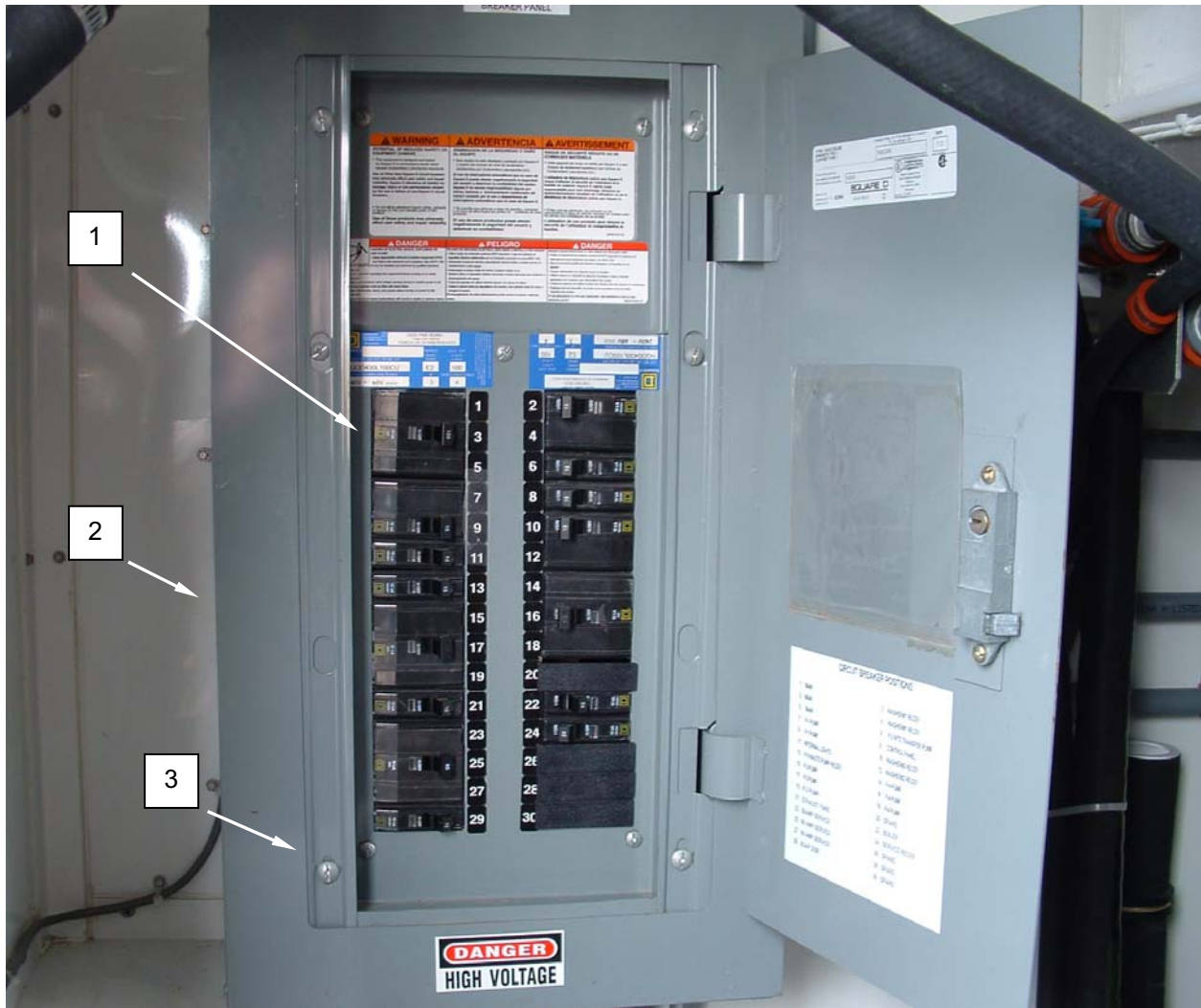
Figure 1. Test Circuit Breakers – Main Panel.
