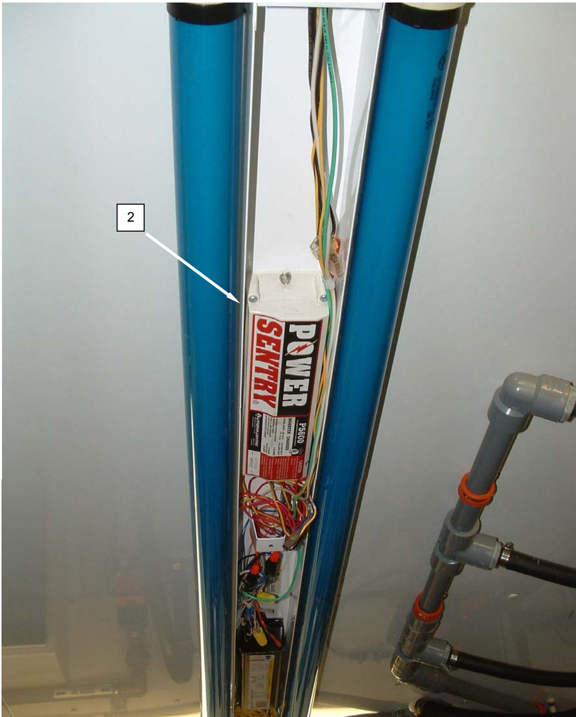
Figure 2. Replace the Battery.
